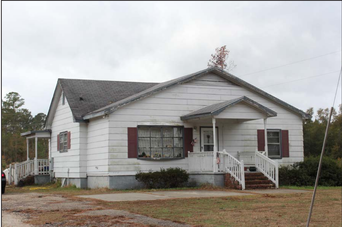
Photo 10. CD1467, facing southwest.
