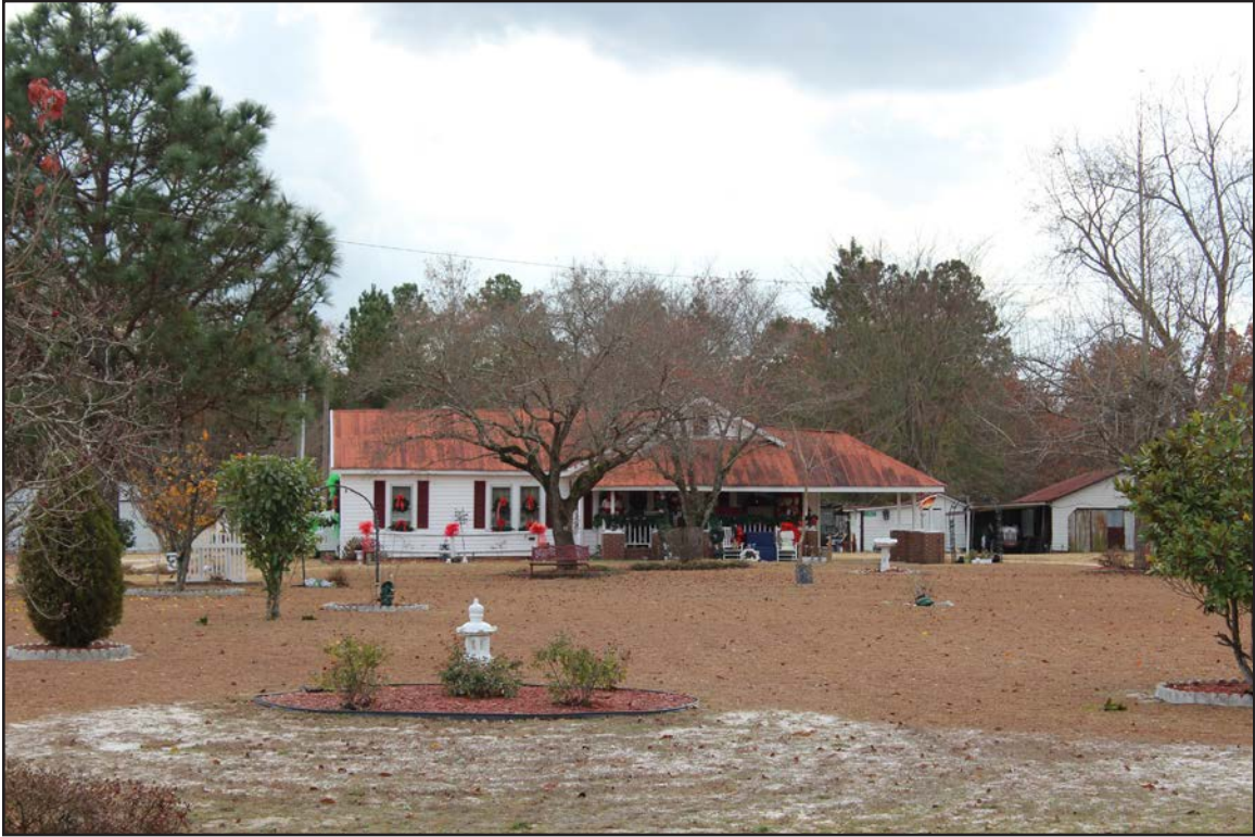
Photo 21. CD1470, facing southwest.
