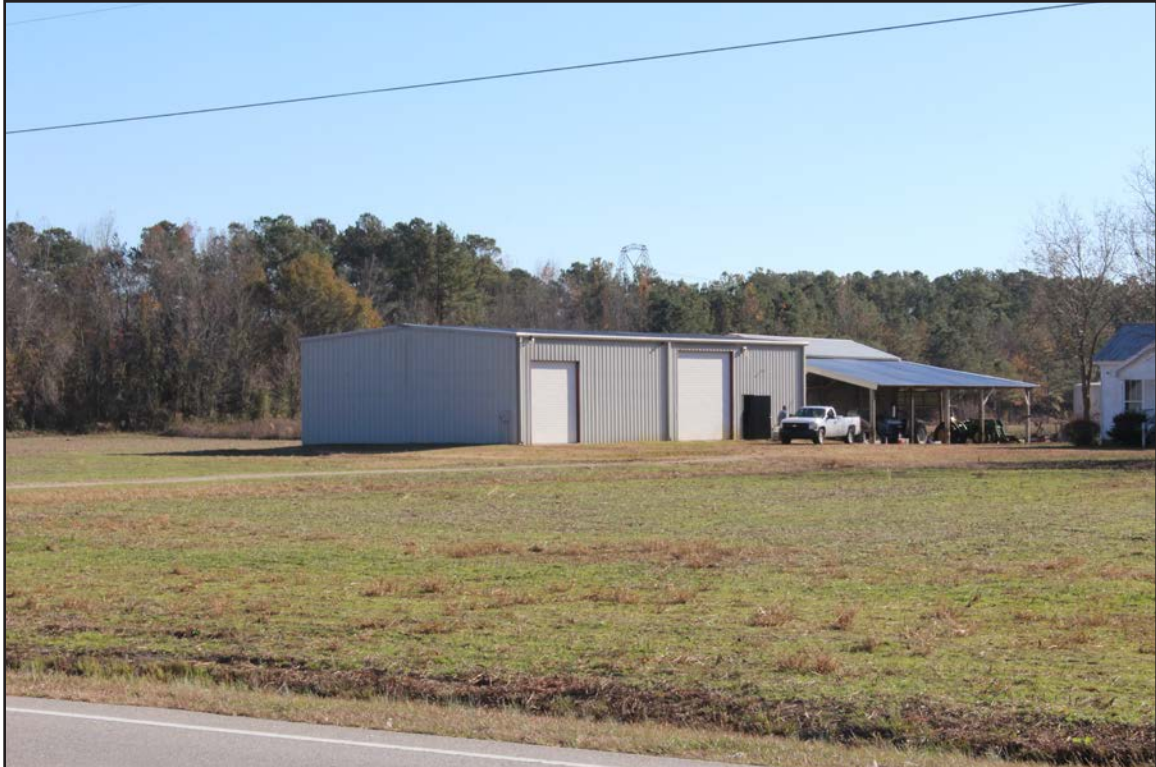
Photo 34. CD1473, storage buildings, facing south.
