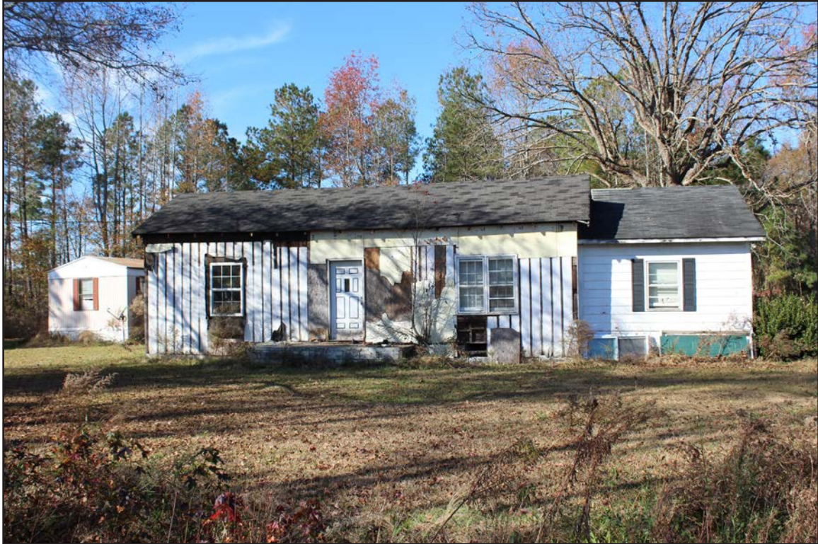
Photo 42. CD1476, facing northwest.
