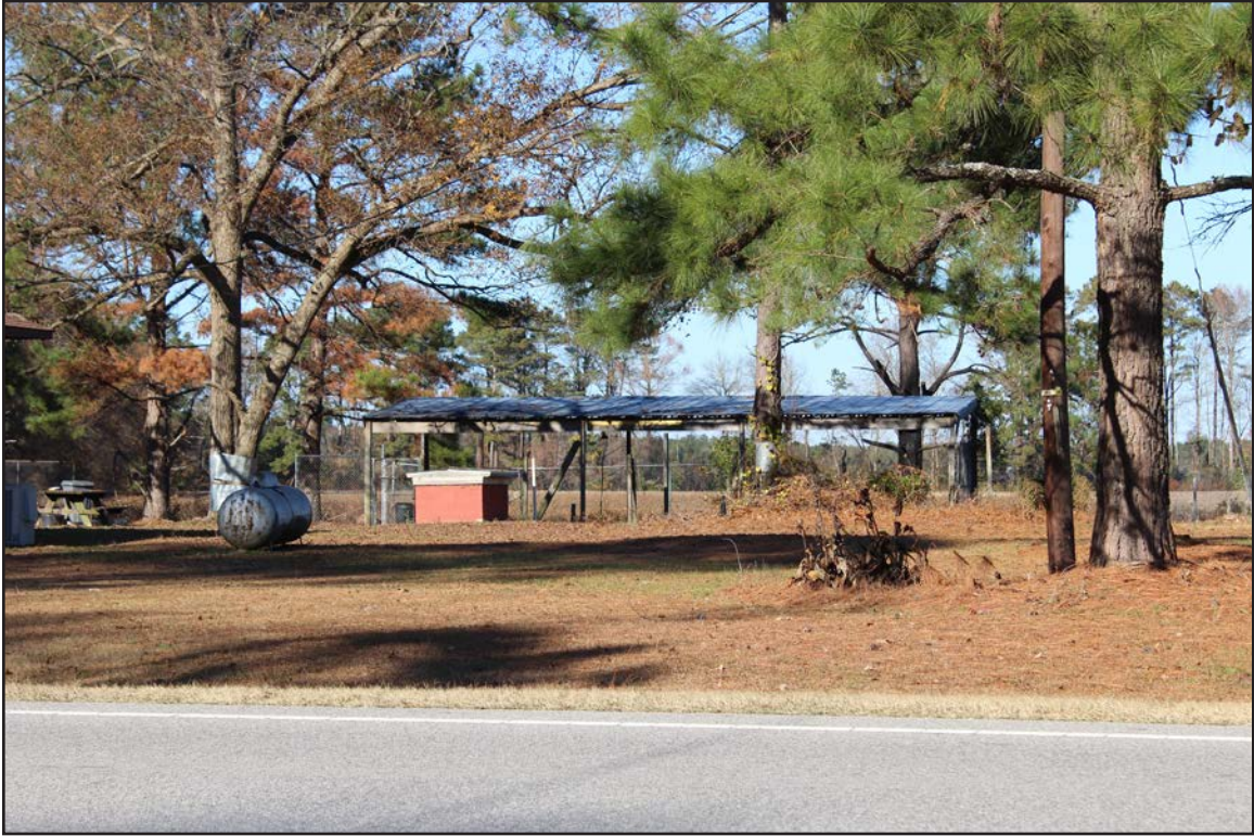
Photo 37. CD1474, well and open air roof covering, facing north.
