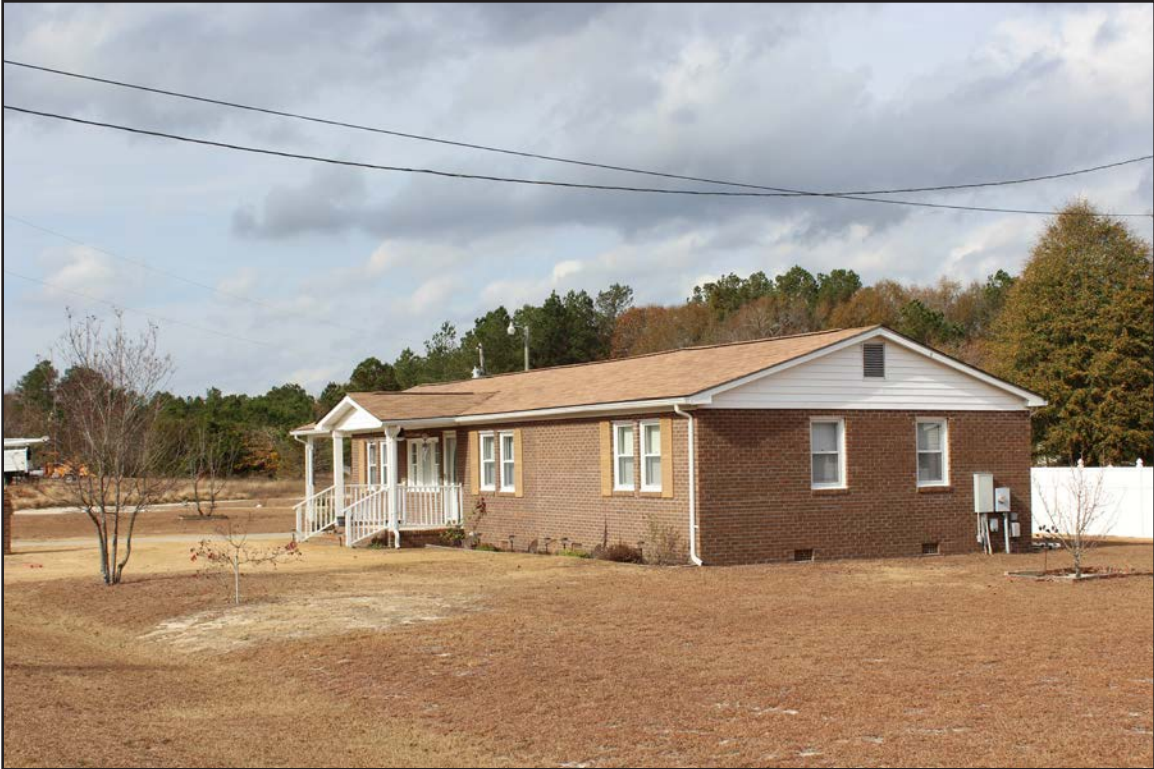
Photo 18. CD1469, facing north-northwest.
