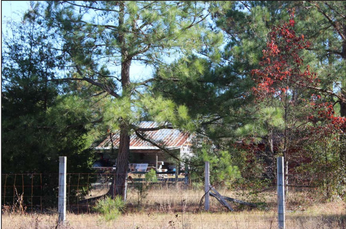
Photo 28. CD1471, shed, facing east-southeast.
