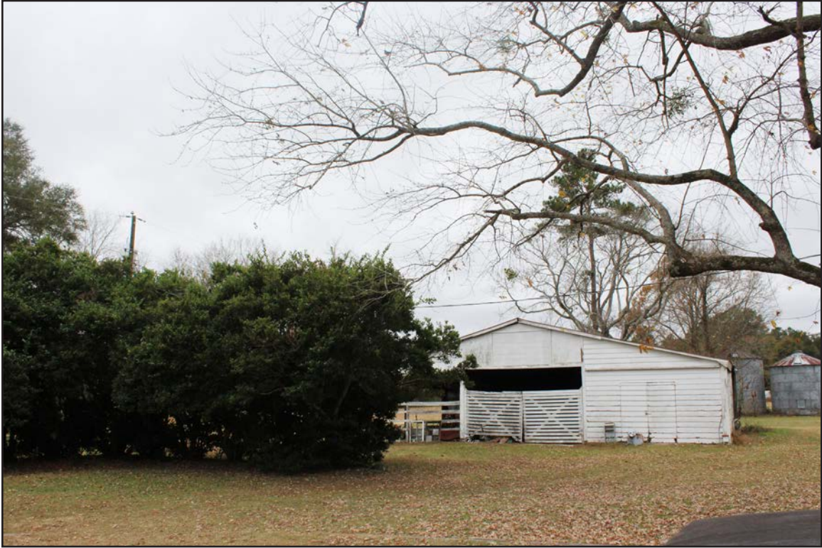
Photo 5. CD1465, Outbuilding 4, facing northwest.
