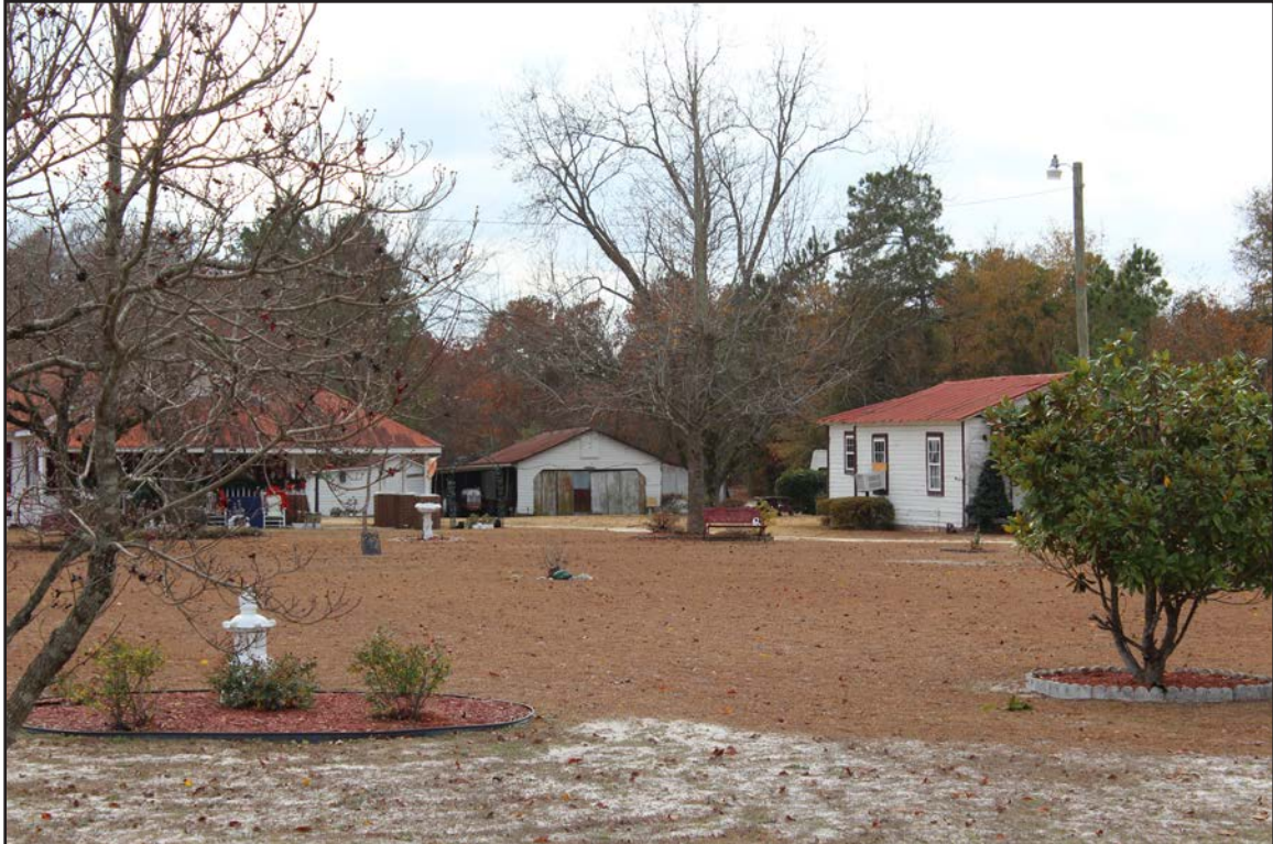
Photo 22. CD1470, garage, facing west-southwest.
