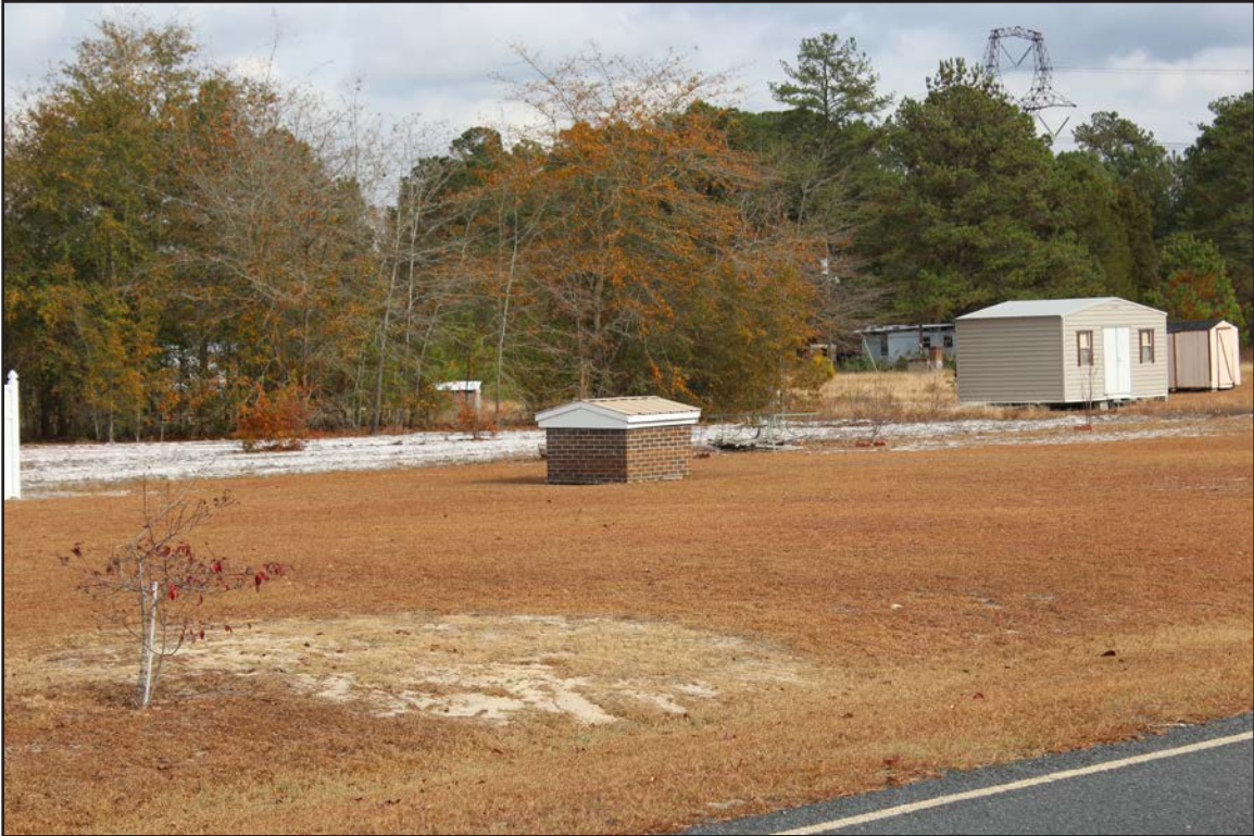
Photo 20. CD1469, well house, facing east.
