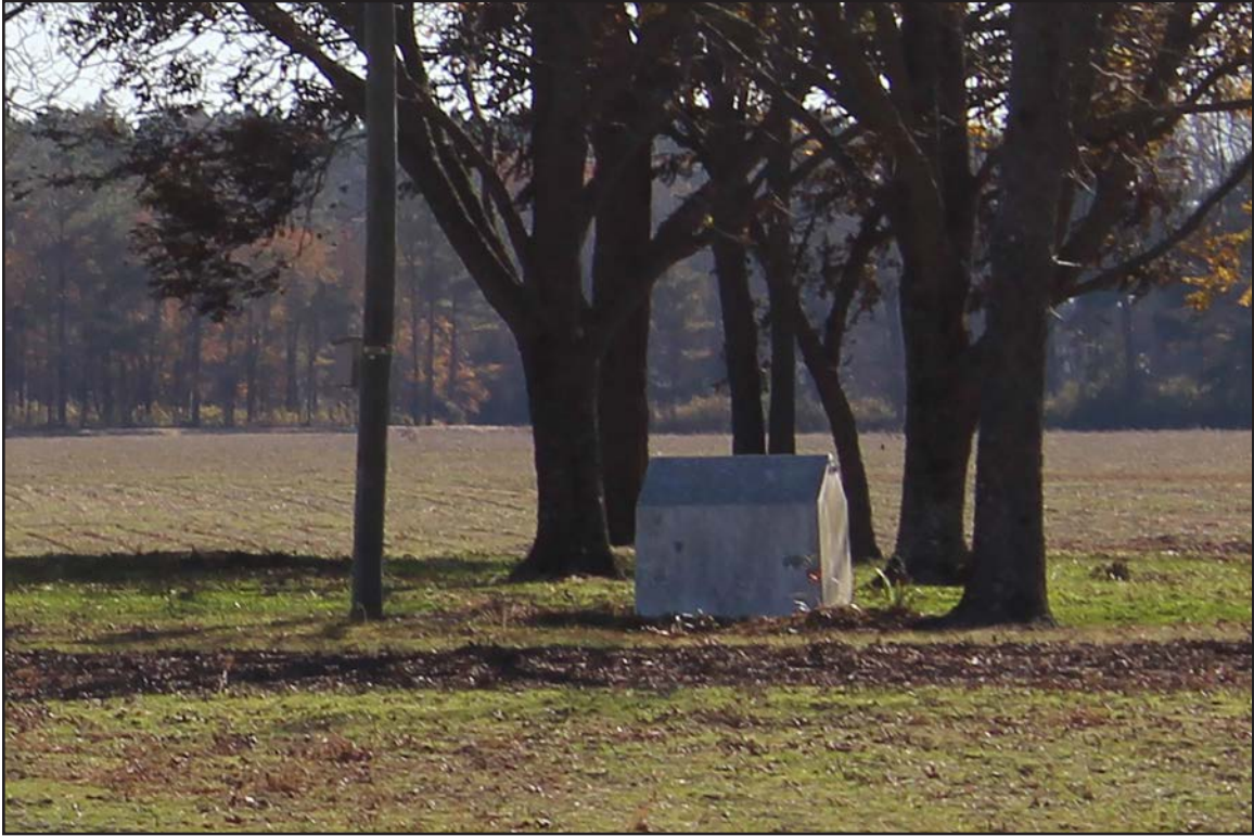
Photo 33. CD1473, well house, facing south-southwest.
