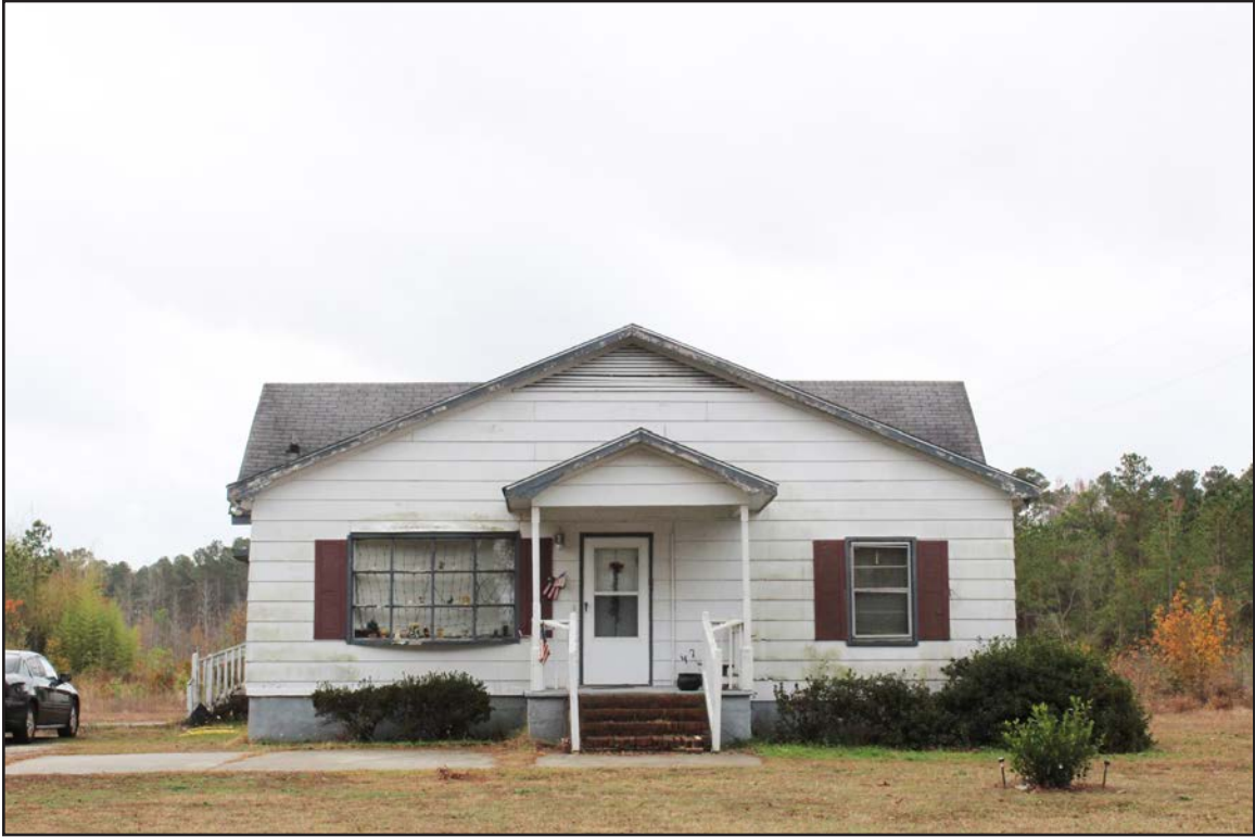
Photo 9. CD1467, facing south.
