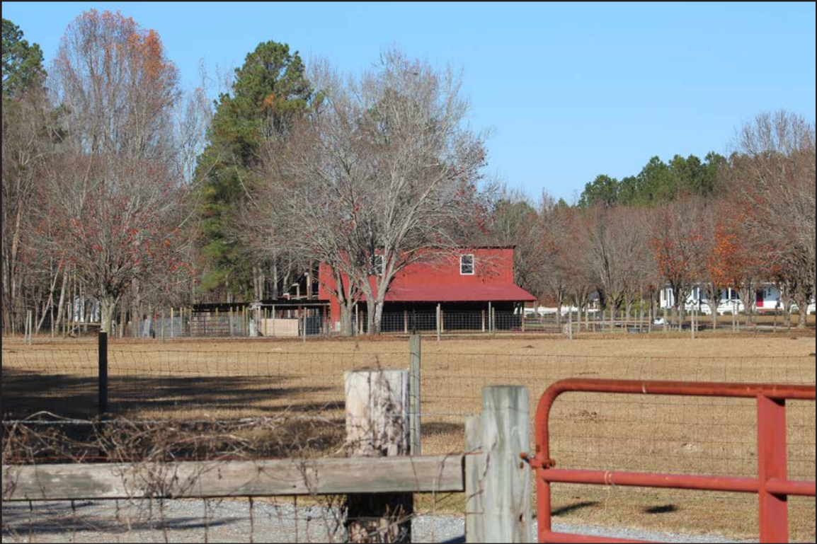
Photo 31. CD1472, barn, facing north.
