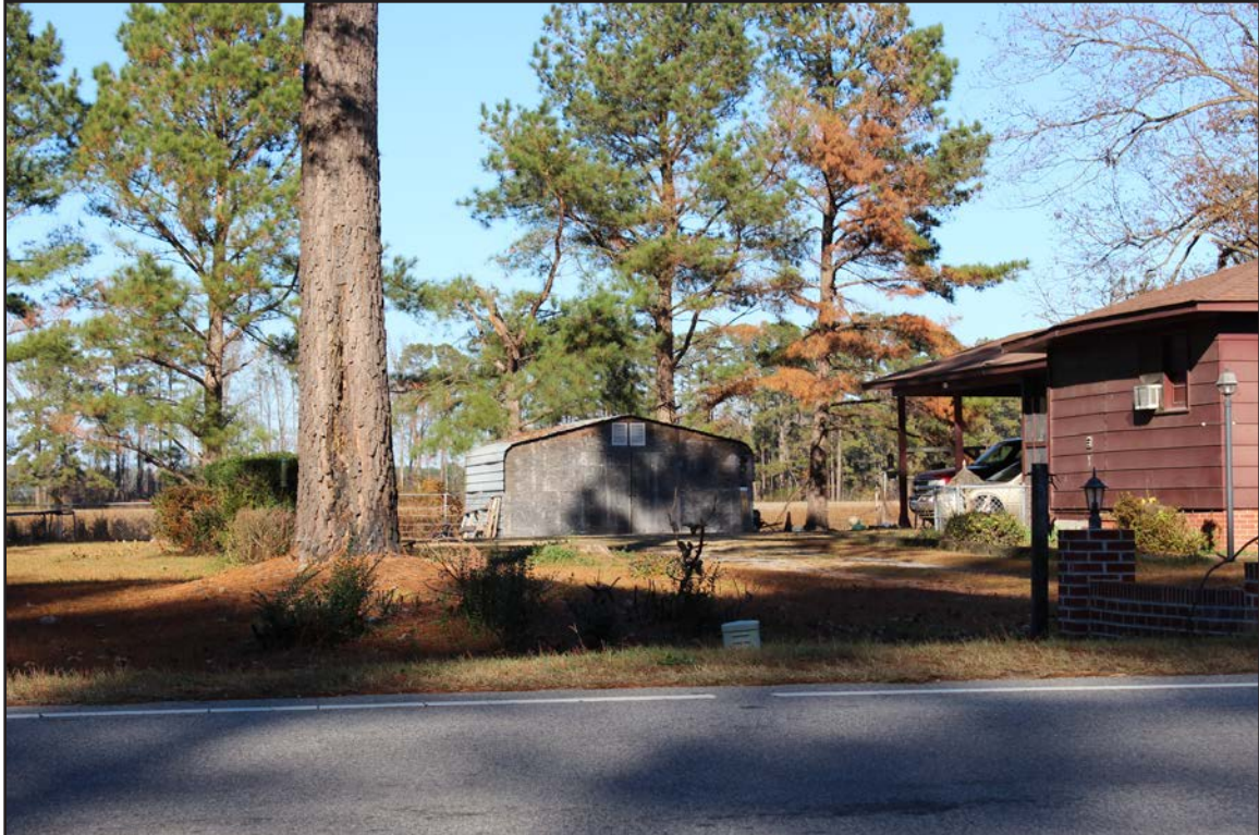
Photo 38. CD1474, parking structure, facing northeast.
