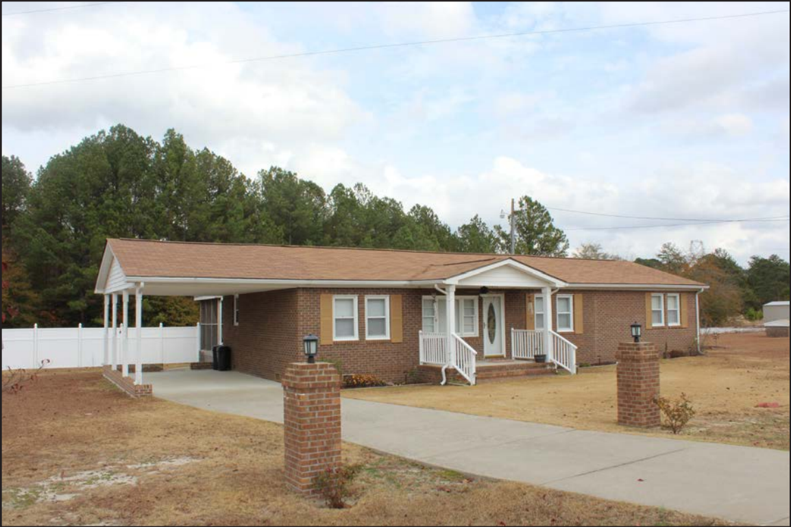
Photo 17. CD1469, facing east-northeast.
